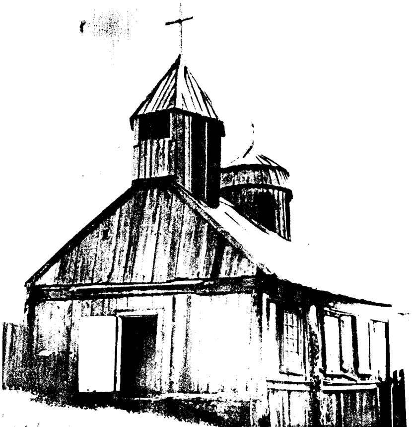
The Chapel following George W. Call's restoration in 1899. Note repair of roof area and replacement of broken windows. The original wooden lectern and candelabra can be seen to the left of the door.
