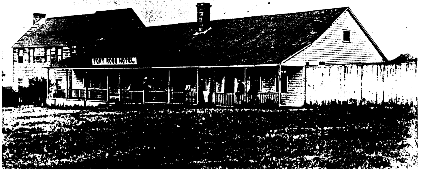
FORT ROSS HOTEL (ROTCHER HOUSE WITH TWO STORY BENITZ ADDITION) 1880
