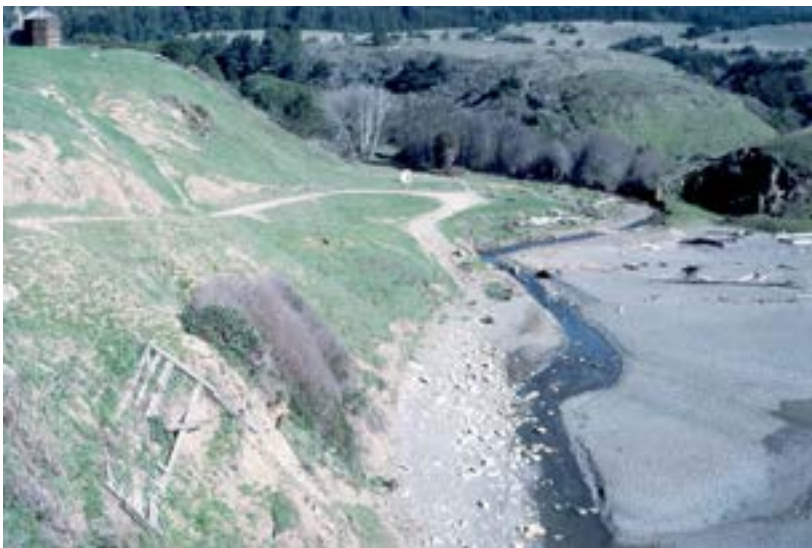
Figure 4-1: Project Area, View Northeast
