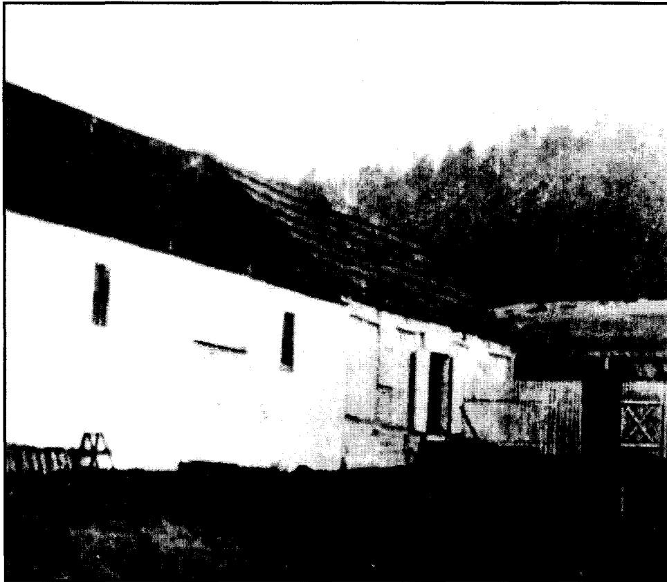
Figure 10. Old Magazin (?) with adjacent building, ca. 1866.
