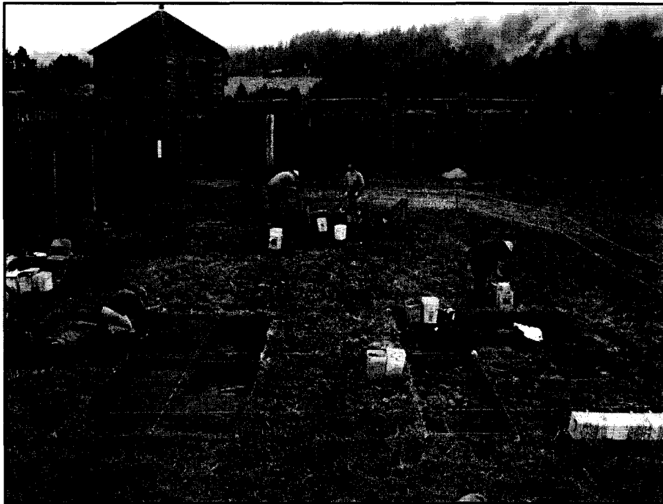
Figure 20. Overview of New Magazin excavation, 2003. View to the north.
