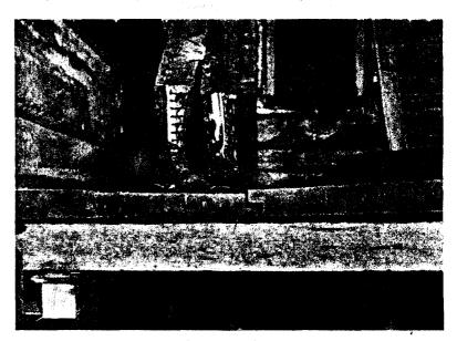
Some partitions reseted directly on the flooring and the doors frames were tenened into the floor. The presence of the old mortis scars. may assist in locating some of the original partitions.
