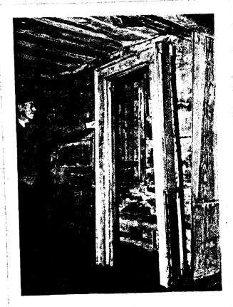
This figure shows the detail of the joining of the sides and header of both dose she widow frame. Note the groove and the bevel shown. The header is on the right. The typical mottis and tenen joint is seen center.
