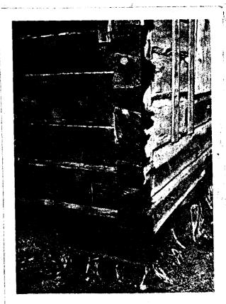
The picture here gives some idea of the key and dove-tail cut. This view shows the painted inside surface of a wall log and it lower surface detail. The notch to the left of the card is the narrow end of the wedge cut to receive the key in the nex log.
