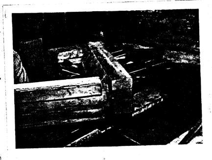
This shows an original window frame in place with the old molding. The sill has been cut through in later mutilation. Note the deep bevel. There is a 1½ in. rabbit on the outside which forms the window jam. All joints are moris and tenemed. The header issecured by the wide shim which shows above the top molding.
